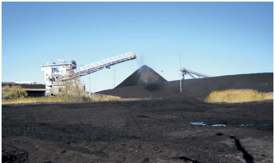
Coal Pile Unloading
