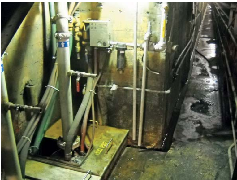
Conveyor Upgrade Sumps
